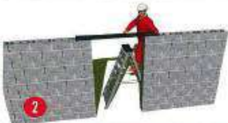
2 Lintel is placed in position
