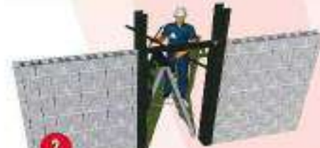
2 Commencement of lintel form work
