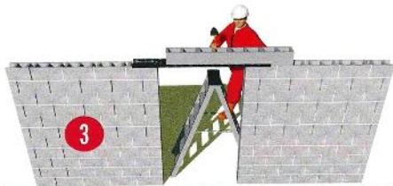
3 Continuation of block work can be carried out immediately
