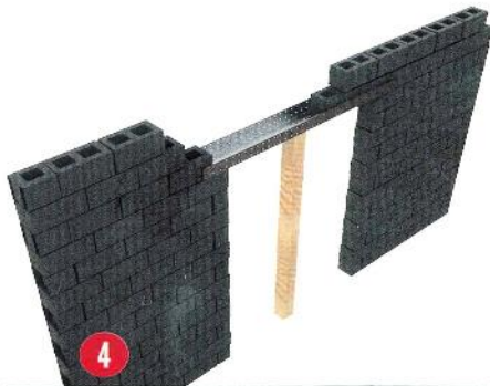
4 Before laying the blocks down on lintel, place a temporary support beneath the lintel to provide support and to prevent deflection. Temporary support can be removed after the mortar sets, (approximately in 3 to 5 hours).
