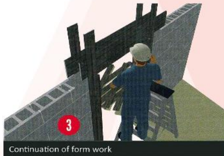
3 Continuation of form work
