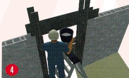
4 Completion of lintel after steel reinforcement and pouring of concrete
