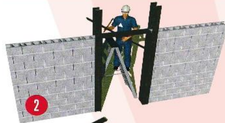
2 Commencement of lintel form work
